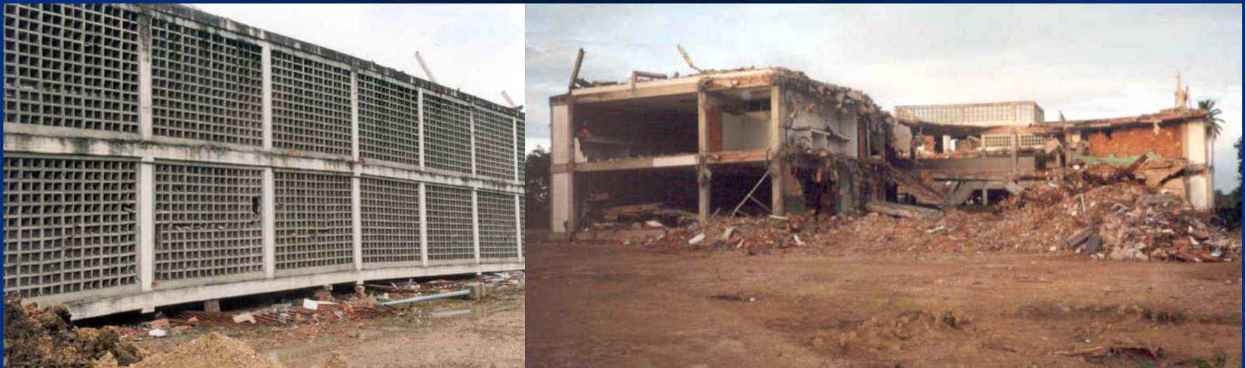
Collapse of an undergraduate school building in Cariaco, Northeastern Venezuela (July 9, 1997)
